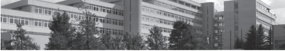
Picture 3. The Educational Departments' Buildings of the Armed Forces Academy of General Milan Rastislav Štefánik (AFA) in Liptovský Mikuláš
